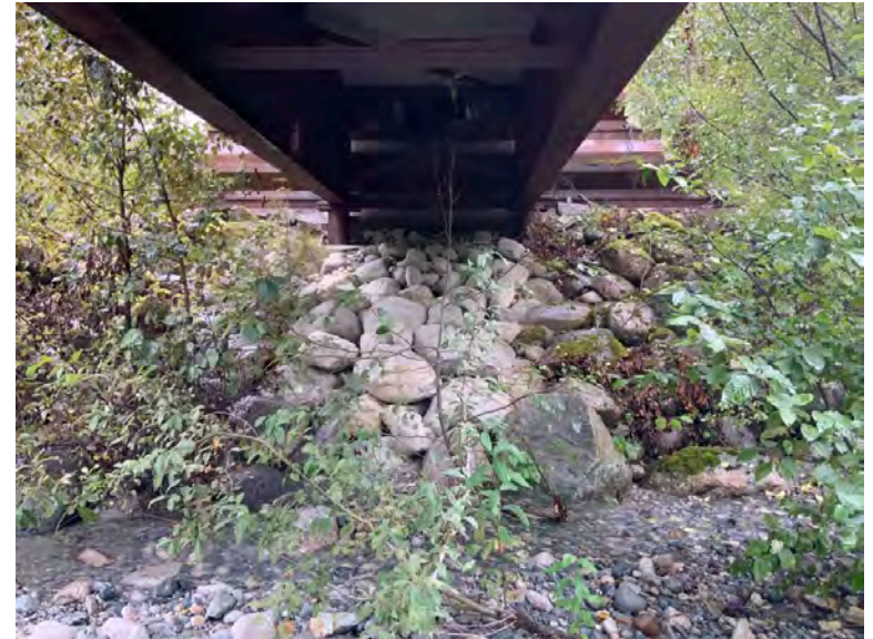
Right Bank Abutment when facing downstream
