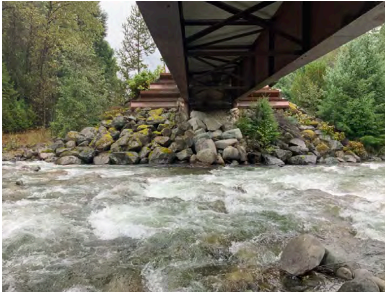
Left Bank Abutment when facing downstream
